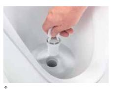
A trap adapter opens the drainage access.
